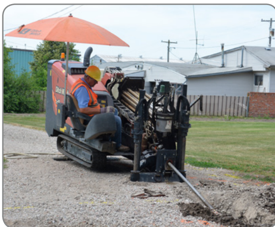
Hamilton crew members boring conduit for fiber under the street.
